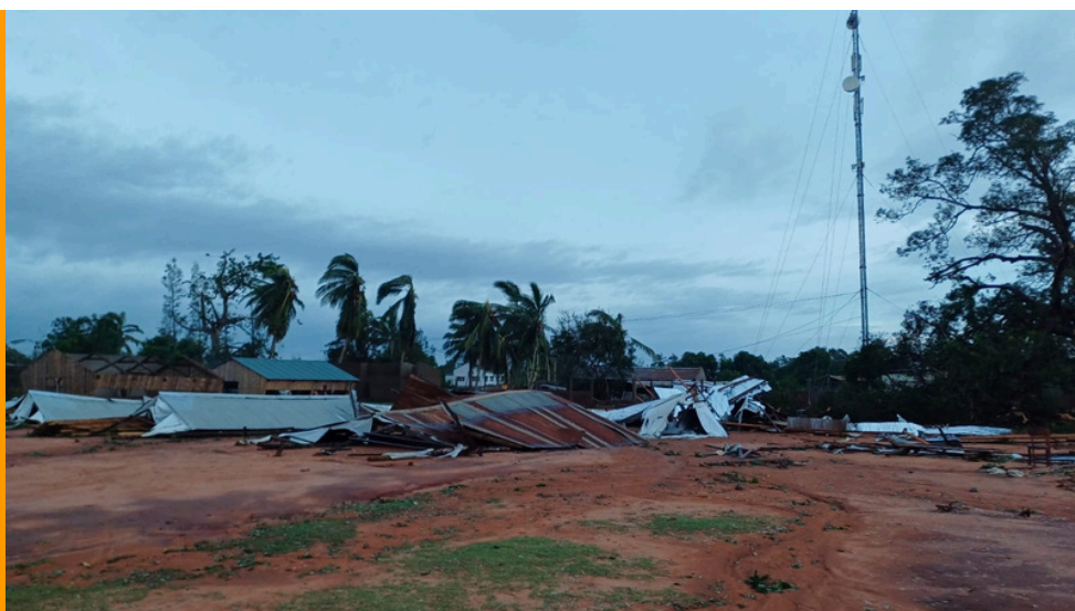
Chiuro Primary School after Cyclone Chido hit in December 2024 (Credits: WeWorld)
