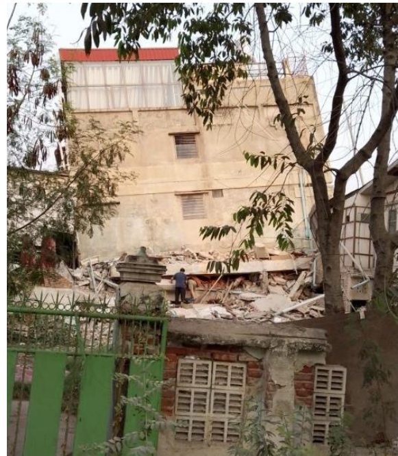
Damage in Mandalay Photo credit: Child Development Association
