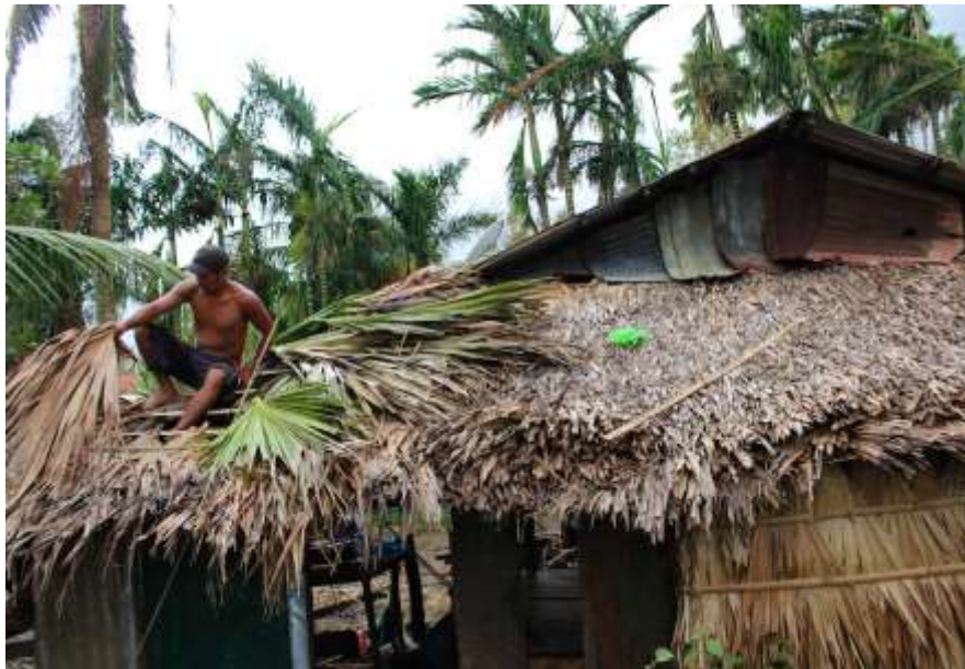
Photo: A father repairing the roofing of their damaged house.
