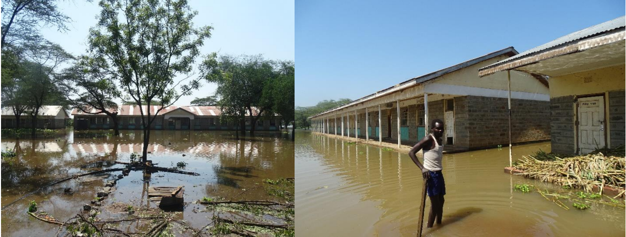
Classroom at Salabani Secondary School Flooded
