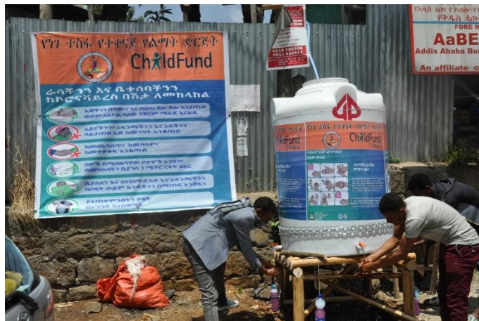
Figure 1 Sample picture taken from Hand Washing facility installed at one community in Arada Subcity -AA. Curtesy to FHIDO
