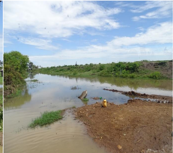
(Left) Access roads Flooded in Kisumu County
